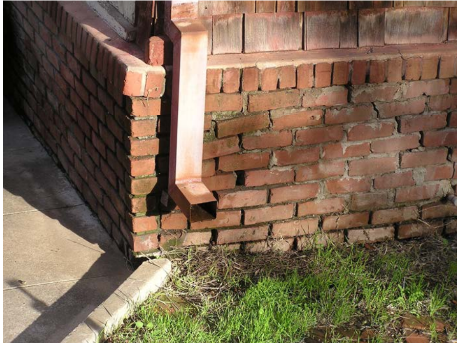
Photograph #9: Deteriorated Mortar in Brick Veneer
