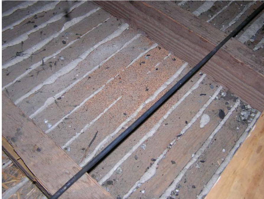
Photograph #1: Signs of Termite Activity
