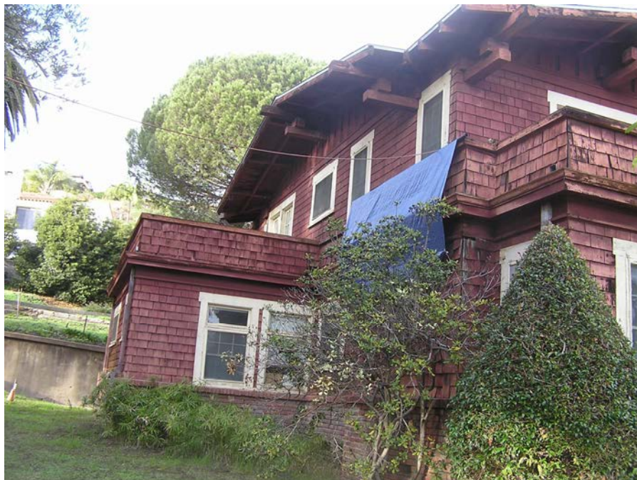
Photograph #10: Tarp on West Side
