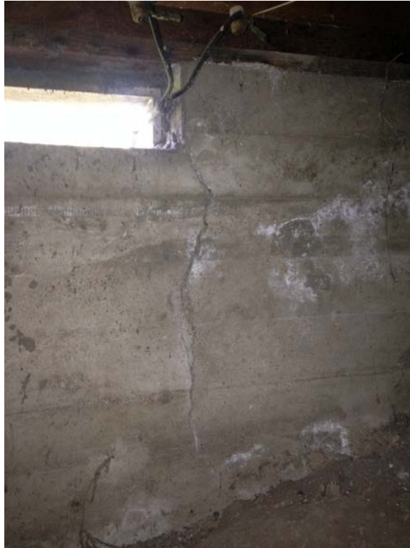
Photograph #5: Crack In Foundation Wall On South Side
