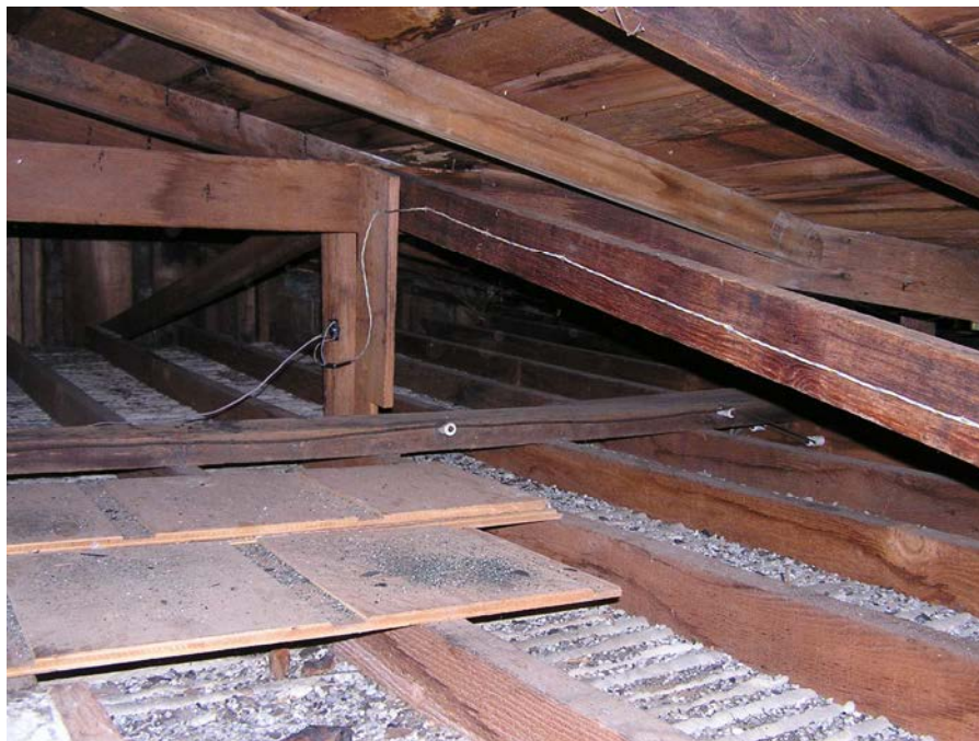
Photograph #2: Deflected Second Floor Ceiling Joists
