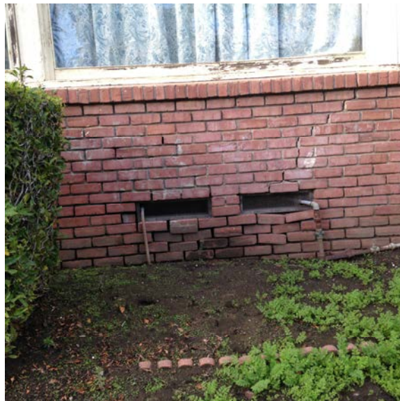
Photograph #6: Cracked Brick Veneer at Southeast Corner
