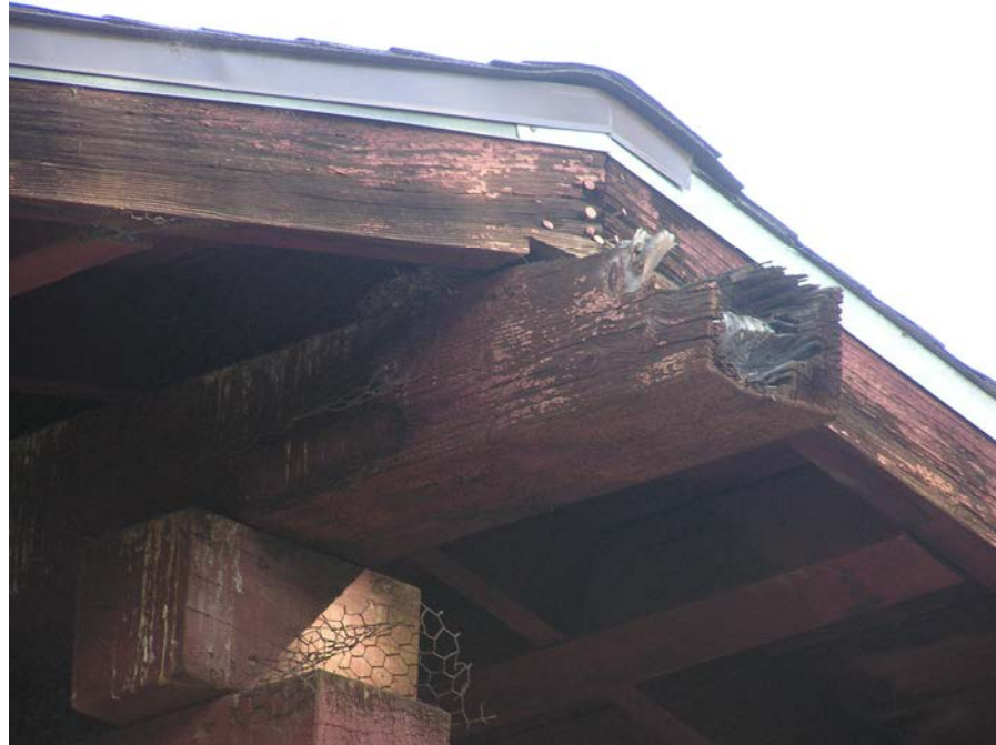
Photograph #7: Damaged Exposed Wood Framing Below Roof Overhang
