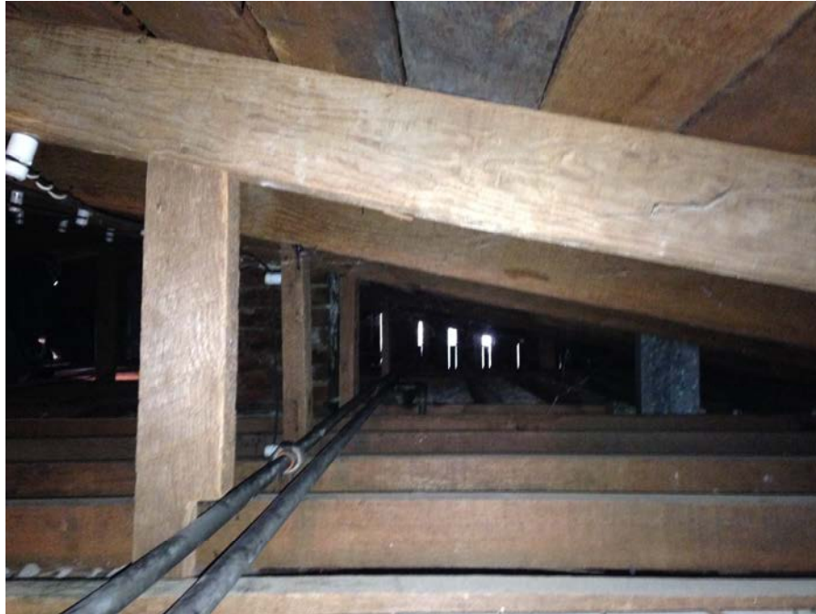
Photograph #3: 2x4 Stud Supporting Roof Rafter
