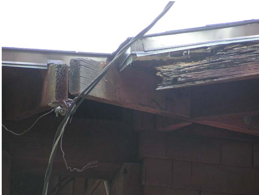
Photograph #8: Damaged Exposed Wood Framing Below Roof Overhang
