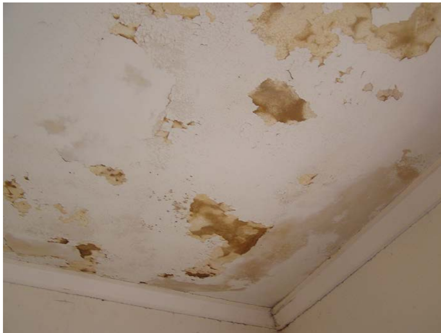
Photograph #4: Stained Ceiling at First Floor Below Exterior Balcony
