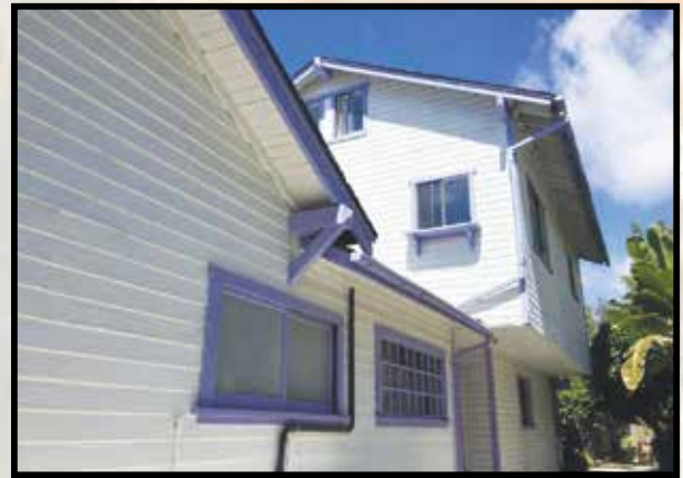
Cottage + attached 2-story addition
