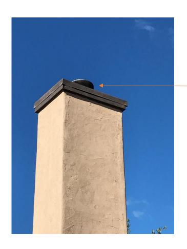
The fireplace does have spark arrestor rain cap.
