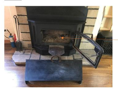
The fireplace has a wood burning insert installed.
