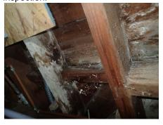
**101:** The posts and piers do not have positive connections, such as T-straps or Teco clips. These are required by current codes, but may not have been when this structure was built, and you may wish to have a specialist comment.
