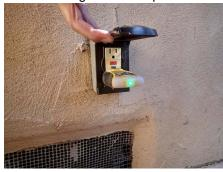
**47:** - Bubble type covers are recommended for permanently installed exterior components because they are more resistant to moisture.
