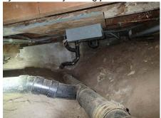
161: - Improperly supported pipes. Metal straps, are substandard but not uncommon.
