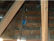
298: - There are open electrical junction boxes, which should be sealed to contain any arching or sparking that might occur.
