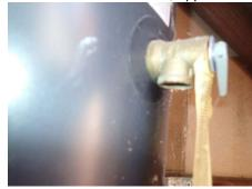
149: - The discharge pipe from the pressure relief valve has been incorrectly plumbed uphill. This is not correct and the discharge pipe should be correctly plumbed.
