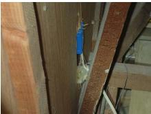
**300:** - Obsolete and suspect knob and tube wiring is present, which should be inspected and certified as safe, or replaced by a licensed electrician.
