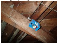
107: - Obsolete and suspect knob and tube wiring is present within the crawlspace, which should be inspected and certified as safe, or replaced by a licensed electrician.
