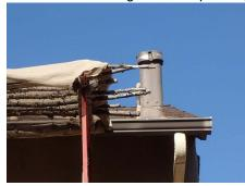
324: - There is no visible wall flashing. We recommend the further review, advice and services of a roofing contractor.
