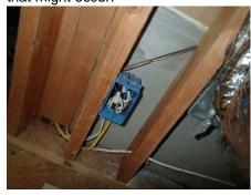
299: - Electrical conduits were not professionally installed, and include detached electrical junction boxes, loose or unsecured vinyl conduit, or conduit without restraint clamps, et cetera, which should be serviced by a licensed electrician.
