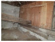
**104: -** The cripple walls have been upgraded to include shearpaneling, and you should request documentation for your records.
