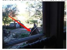
**217:** - Moisture stains and or damage were noted at some window sills. We recommend the further review, advice and services of a window installer/repair person.
