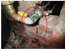
127: - The property was originally plumbed with other water pipes, but most if not all of them appear to have been replaced with copper. You should request documentation, and any warranty or guarantee that might be applicable, which will confirm that the work was done to code and by a specialist, and may include a warranty or guarantee.
