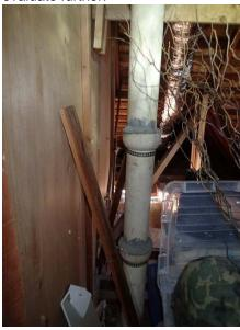
331: - Asbestos like materials were noted at the basement / crawlspace . Identifying asbestos is outside the scope of this inspection. We recommend service and evaluation by a qualified specialist. Any future work should be evaluated with this in mind prior to beginning any work.
