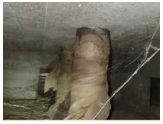
**92:** - Signs of prior moisture that confirm moisture intrusion. While this condition is not uncommon, we recommend the further review, advice and services of a grading and drainage contractor.
