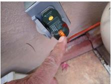
**46:** - A ground-fault protected outlet in the yard does not trip on test, and should be serviced.
