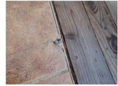
NS 34: - There is an offset or offsets in a walkway that could prove to be a trip-hazard.
