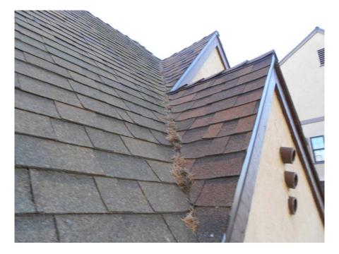
• These appear to be newer shingles and should have step flashing at the roof to wall connection. I was not able to determine that step flashing was used. The roof to wall connection appears to be sealed with mastic.
