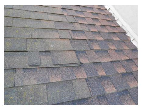
• There are newer shingles over the front entryway and older shingles on the main part of the roof.
