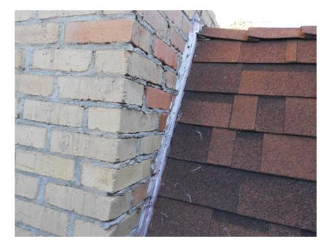
• This photo shows the sides of the chimney. Once again, there is no step flashing or counterflashing.
