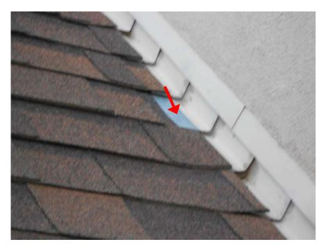
• This photo shows a shingle adjacent to the tie-in where one of the older shingles is cracked.
