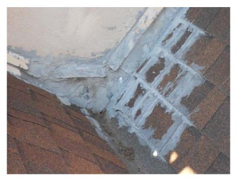
• This photo shows a vent pipe adjacent to the cricket. The seal on this vent pipe appears to be cracking.
