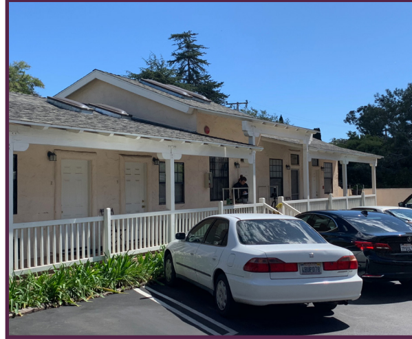
Close-up of west building
