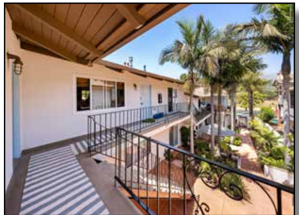
View of Courtyard from Upper Level Walkway
